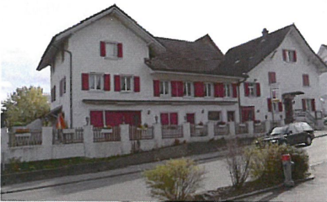
0189 (Nord- und) Westfassade
